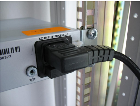
Illustration 4: Angled power cord and earth bonding point
